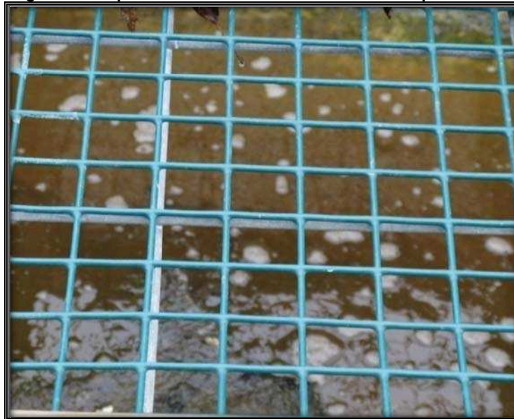
Figure 4: Deep Pool of Feces and Urine Under Occupied Kennel
